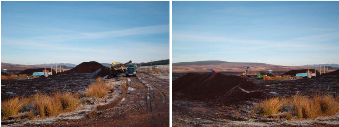
Fig 2 views of existing peat operation on site
